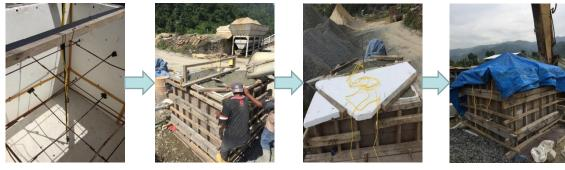
Mock-up Block for Thermal Properties (1.5x1.5x1.5m)
